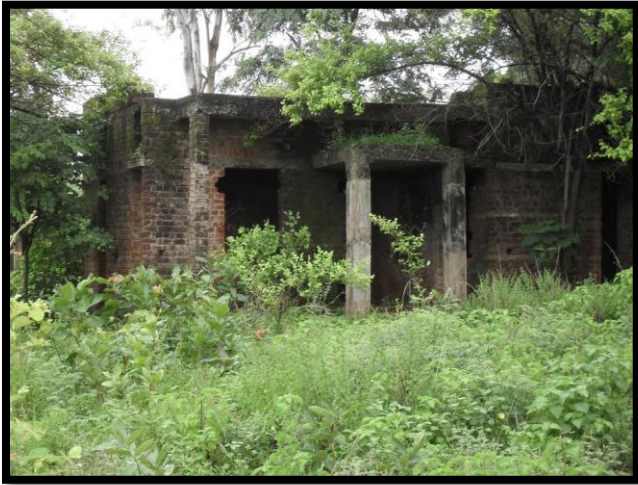
Partially Constructed Quarters
