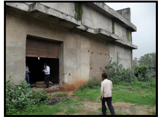
Blow Room Entry Gate
